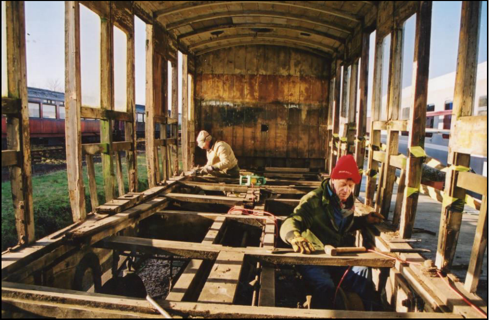
above: In the early days of restoration the work was carried out on no.946 in the open at Ruddington photo: Richard Tilden-Smith
