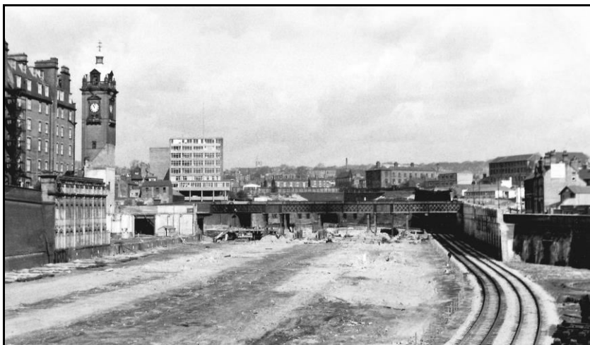
After the demolition of Nottingham Victoria in April 1968.
