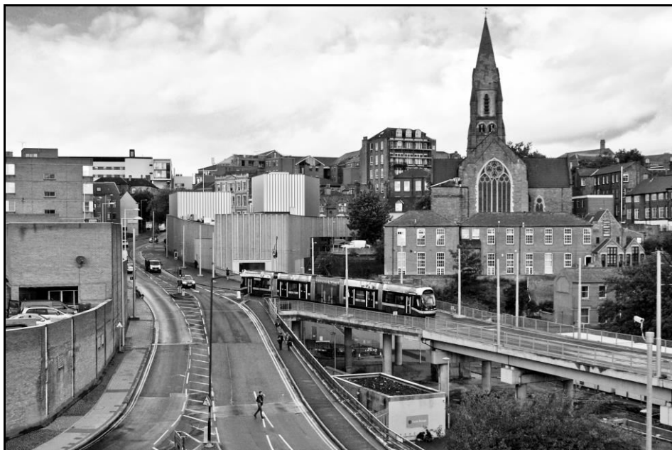
The view from Broadmarsh car park on 4 th October 2013 showing a NET tram making its way from Middle Hill onto the new viaduct that has replaced the GC structure.
